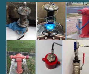
Typical sensing installation alternatives on existing hydrants, pipe taps or air valves
